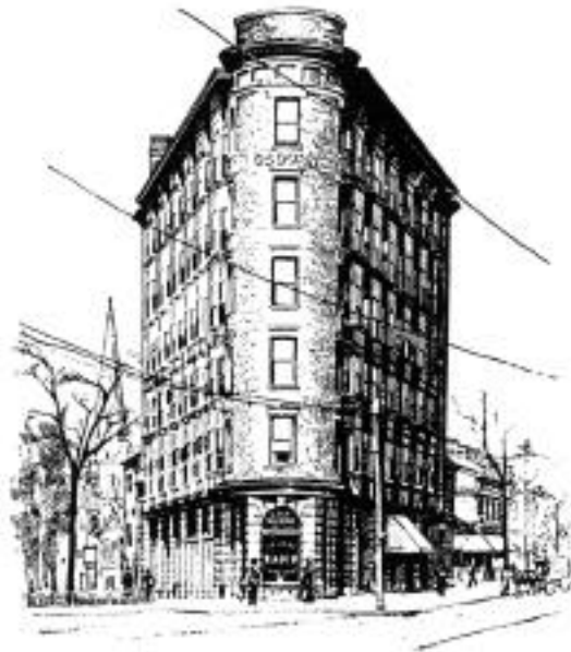
Offices of Drs. Bunts, Crile, and Lower, Osborn Building at East 9th Street and Huron Road, 1897-1920 (artist's drawing)
